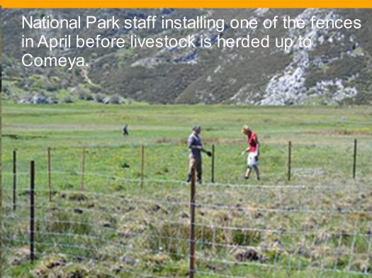
Main fence in Comeya, made of wood and reinforced with wire.
