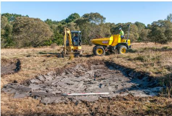
Detail of one of the pools created at the Wetland of Cospeito with the machinery used (small backhoe loader and dumper).
