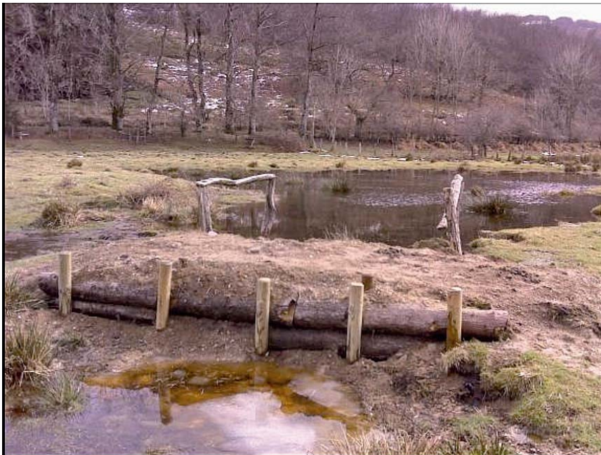
Belate Mire: Recently constructed livestock crossing with right-hand side flooded
