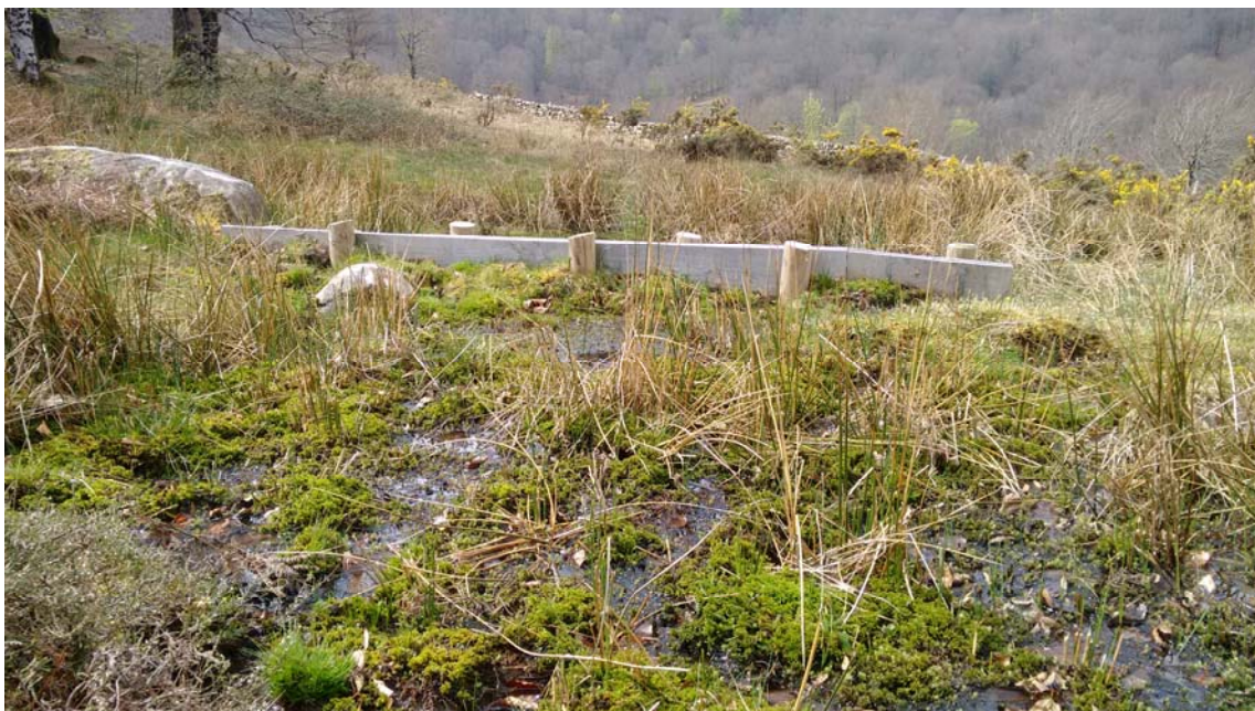
Plant development upstream from the dyke one year after installation.
